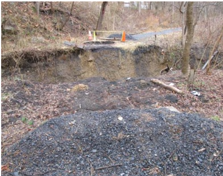
Portion of walking path no longer usable because of excessive stream erosion
