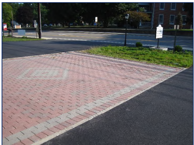
Pervious pavers and rain garden demonstration project at Romney Town Hall.
